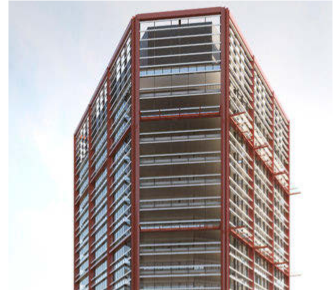
Fig 6.2.50: Side support framed clear glazing to upper fins
