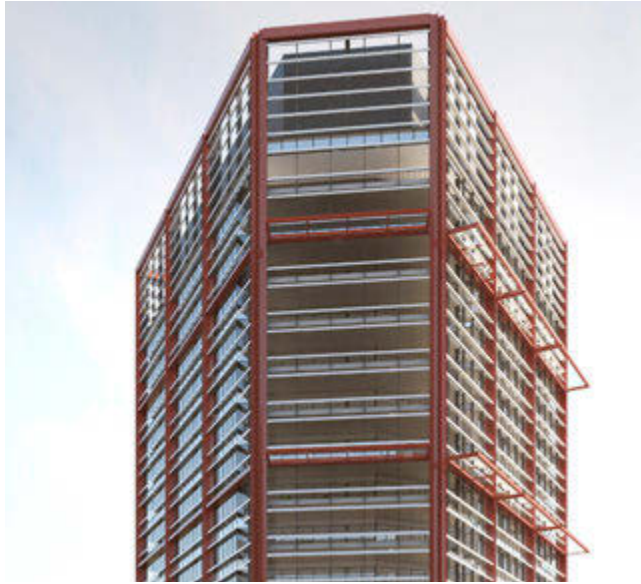
Fig 6.2.49: Framed clear glazing to upper fins
